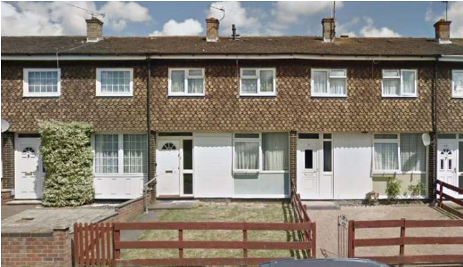
Figure 50. Hexham Road - Hung tiles on front elevations
