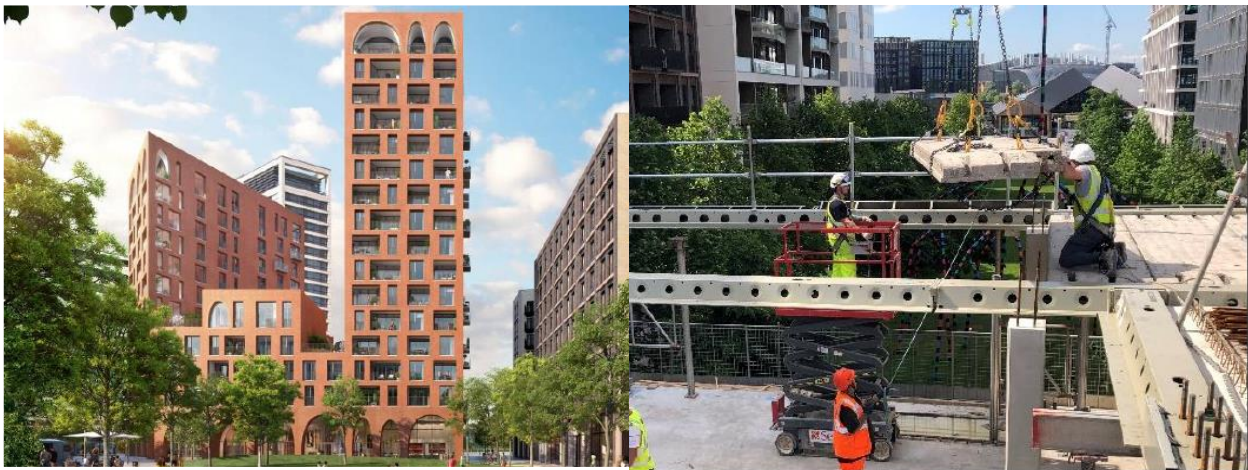
Cadence S5 at Kings Cross by Laing O'Rourke for Argent
