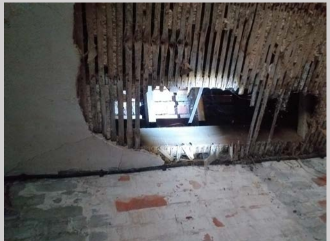
Photograph 6: View of bare tiles of the roof of the southern section of Building 1.
