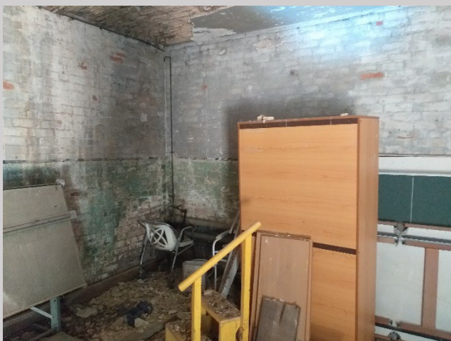
Photograph 7: Example of interior of Building 1
