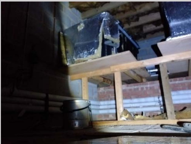
Photograph 19: Inside of roof void/water tank room in Building 3.
