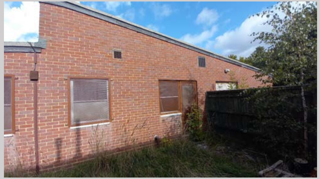
Photograph 12: Southern elevation of Building 3 from the south.
