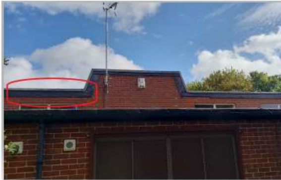
Potential external access point under fascia board, location shown in red.
