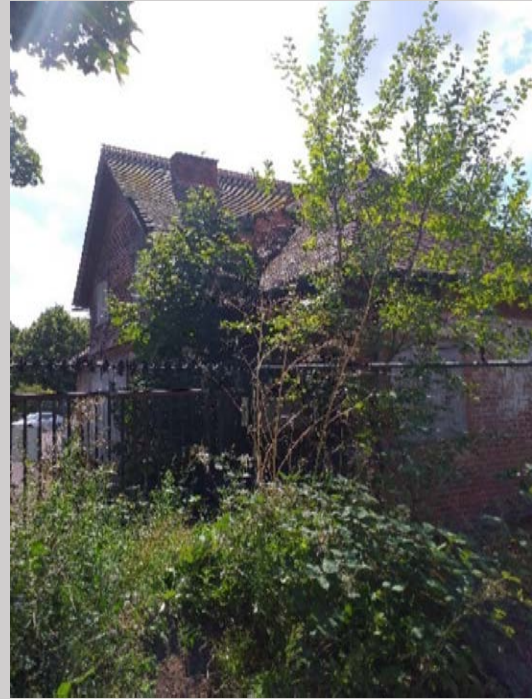
Photograph 2: eastern elevation of Building 1 viewed from the north east.
