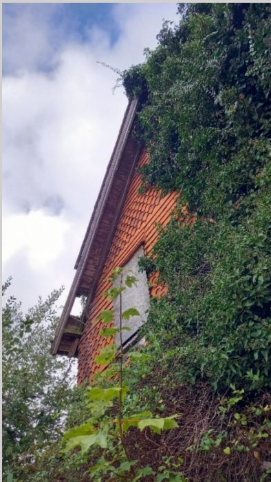
Photograph 3: western elevation of Building 1 viewed from the south west
