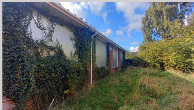
Photograph 9: Northern elevation of Building 2 from the north east.
