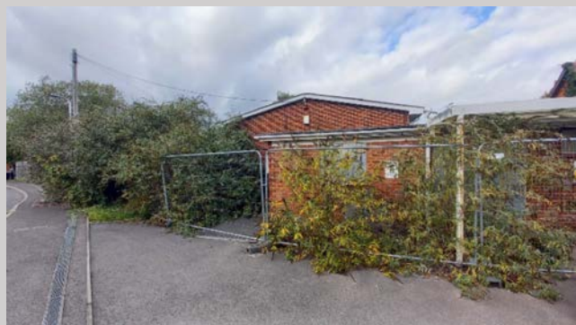
Photograph 8: Southern elevation of Building 2 from the south
