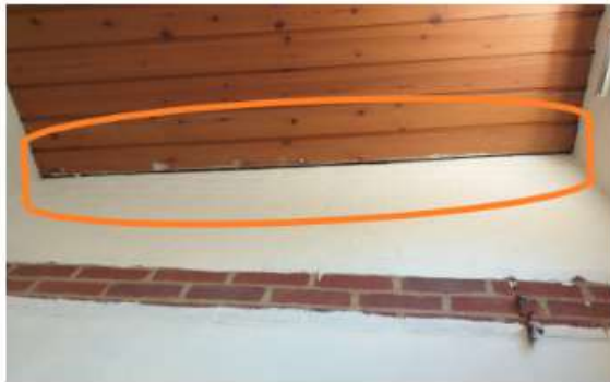
Internal roost feature, gap between wall and wooden ceiling leading to potential space between internal ceiling and external roof. Location shown in orange.
