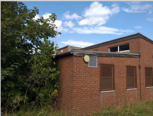
Photograph 13: Western elevation of the southern end of Building 2 from the south west.
