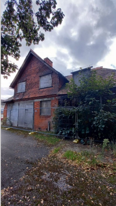
Photograph 1: eastern elevation of Building 1 viewed from the east.
