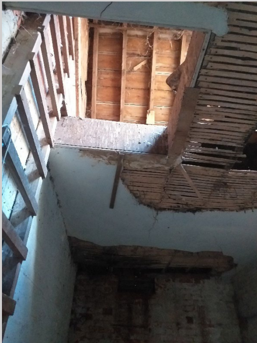
Photograph 5: View of timber cladding lining the roof of the northern section of Building 1
