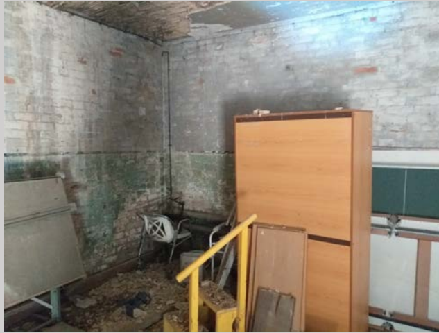
Photograph 7: Example of interior of Building 1
