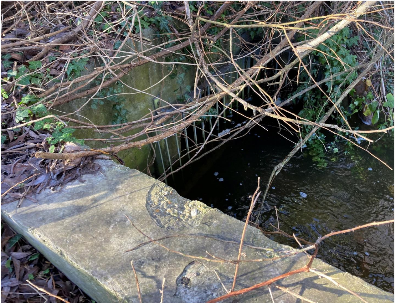
Plate 10 - Culvert exit noted off-Site to the north-east associated with the brook.
