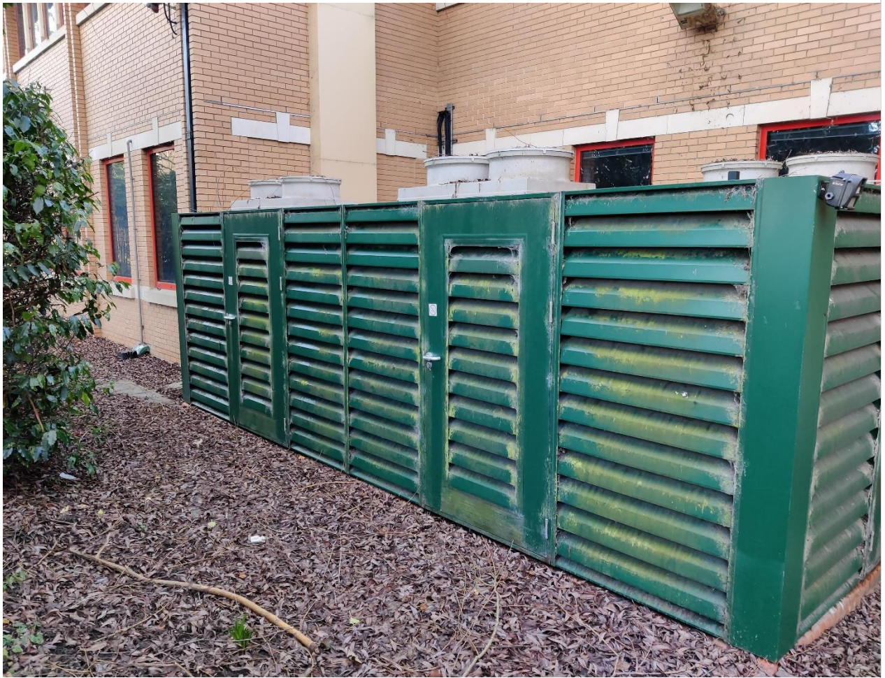
Plate 7 - Green metal unit to the rear of the building on northern part of the Site.
