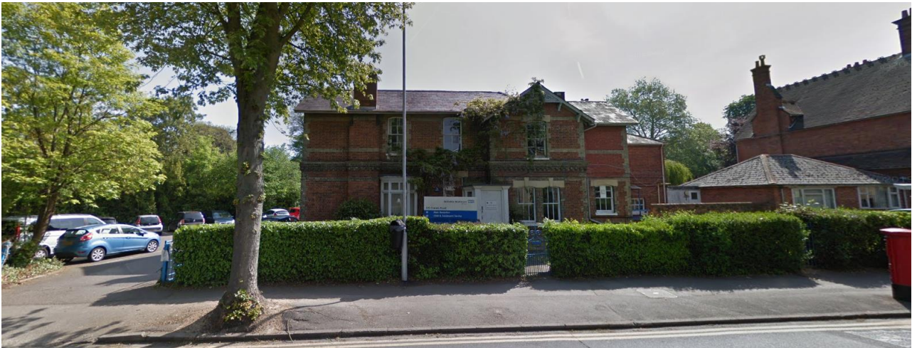
Figure 2. No. 3 Craven Road Streetview (Google Streetview May 2019)
