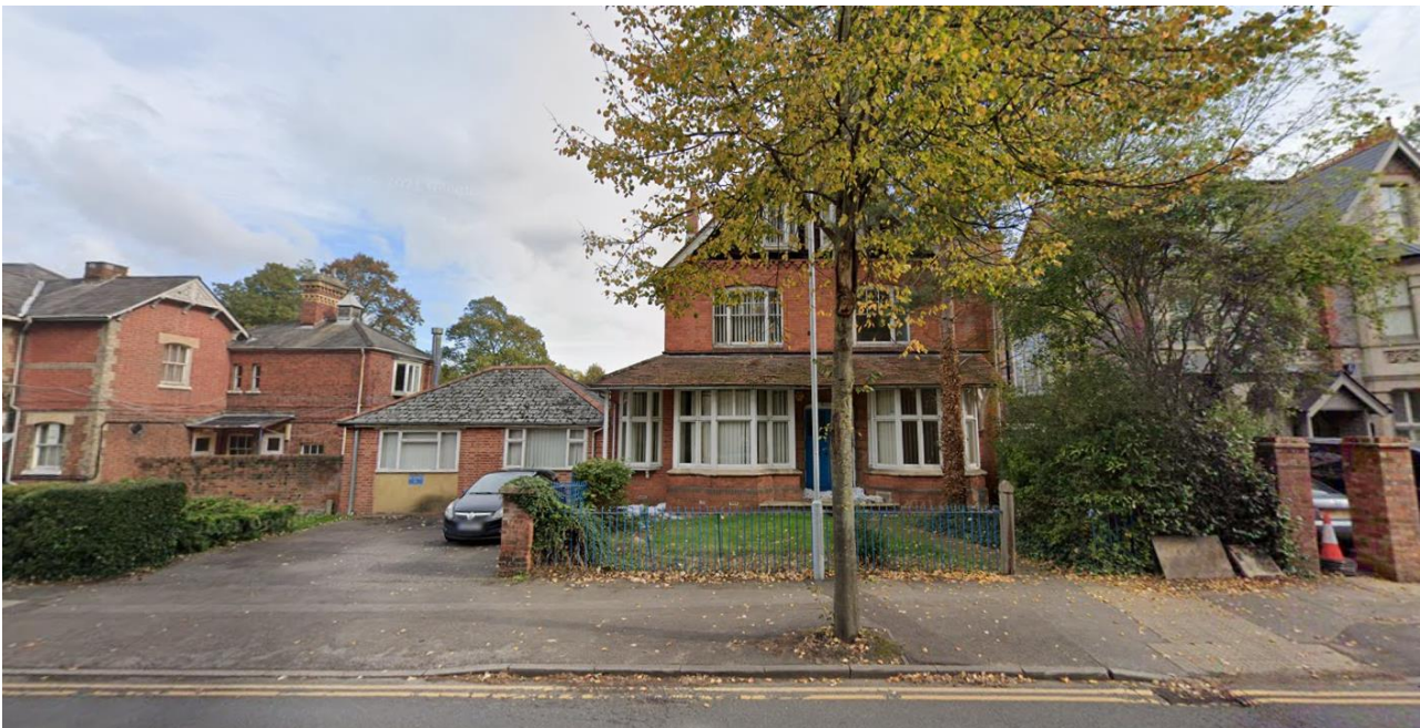
Figure 3. No. 5 Craven Road and link building (Google Streetview October 2020)
