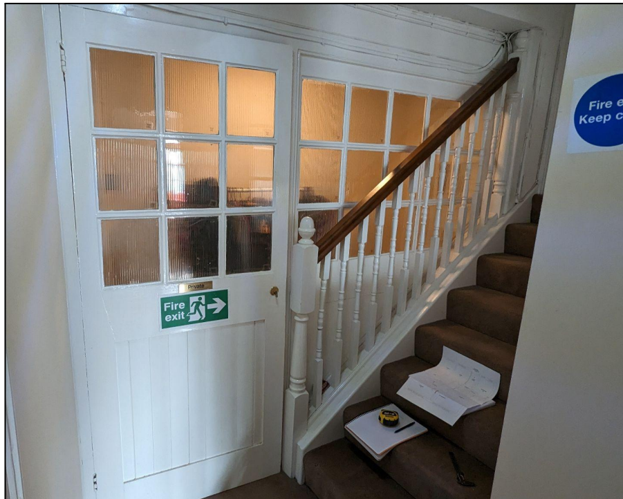
Figure 1: The glazed screen to be altered as part of this Listed Building Consent application.
