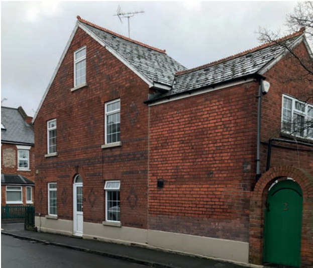
Figure 1-12. A - View towards Site Entrance
