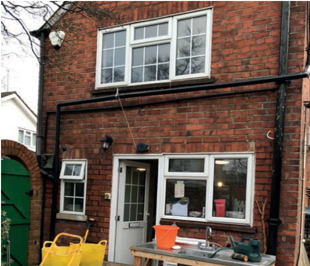
Figure 1-18. G - View toward western elevation
