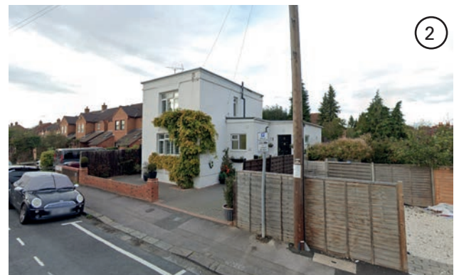
Figure 1-27. Local flatted forms on Gosbrook Road and Montague Street
