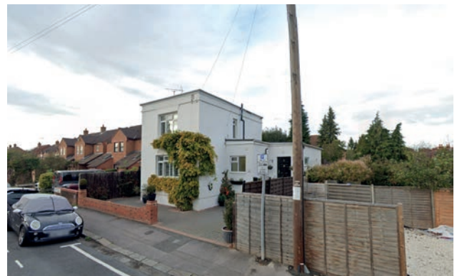
Figure 1-7. View D - 4 Montague Street
