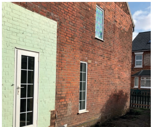
Figure 1-17. F - Lower southern elevation
