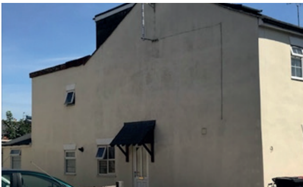
Figure 1-8. View E - Champion Road, adjacent to the site from the north
