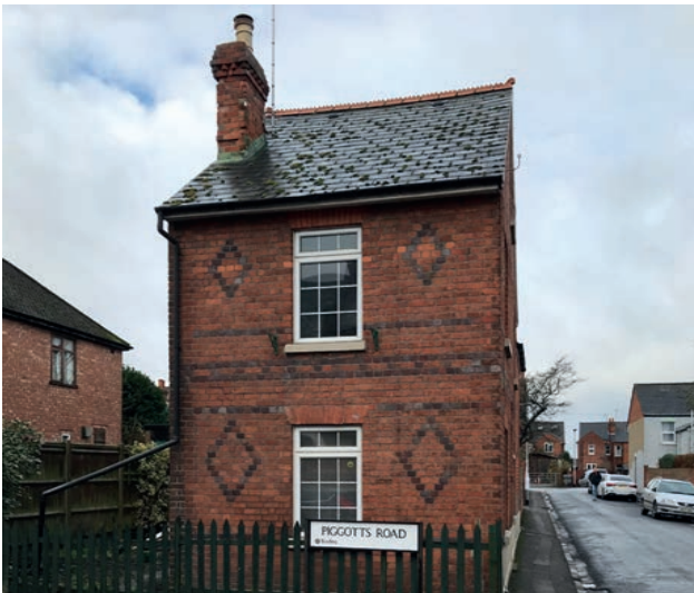
Figure 1-14. C - View towards Rose Cottage from Piggotts Road
