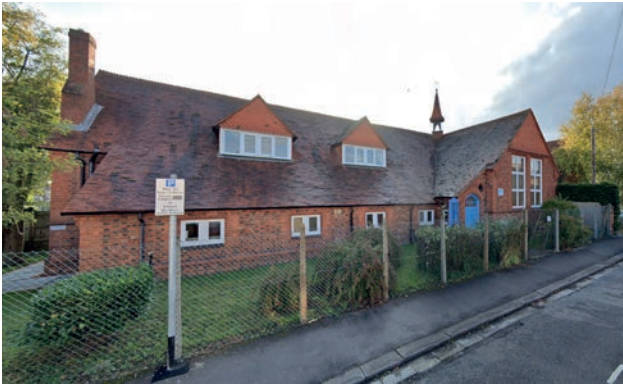
Figure 1-4. View A - Caversham Hall
