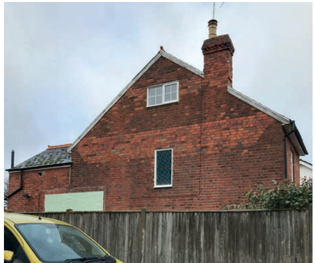
Figure 1-15. D - View towards the southern elevation from Piggotts Road
