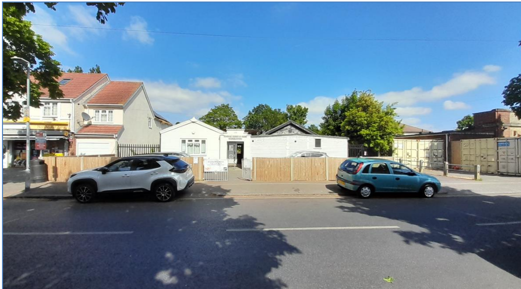
Fig 1. Front of 163 Northcourt Avenue. Photo taken by case officer on 31/05/2023.
