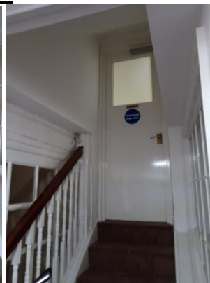
fire escape stairs
