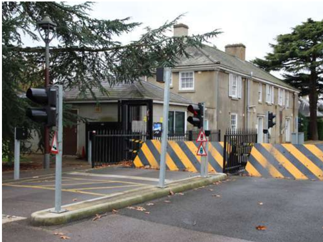
Early twentieth century cottages on Caversham Park Drive will have their settings enhanced.
