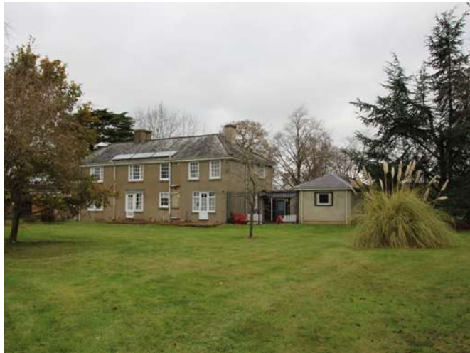
Southern elevations of early twentieth century cottages on Caversham Park Drive.
