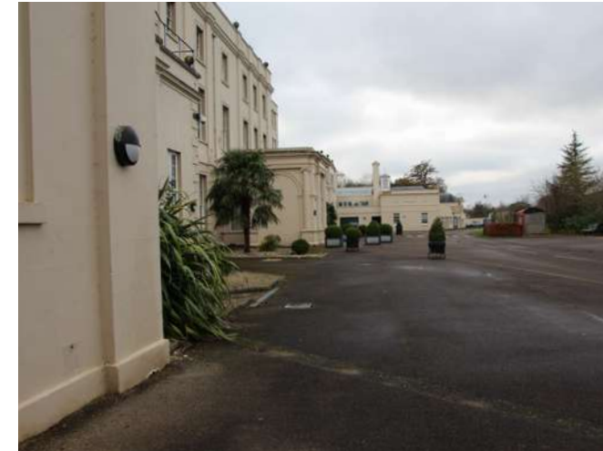
Northern elevation of historic house. Entrance dominated by hard-standing.
