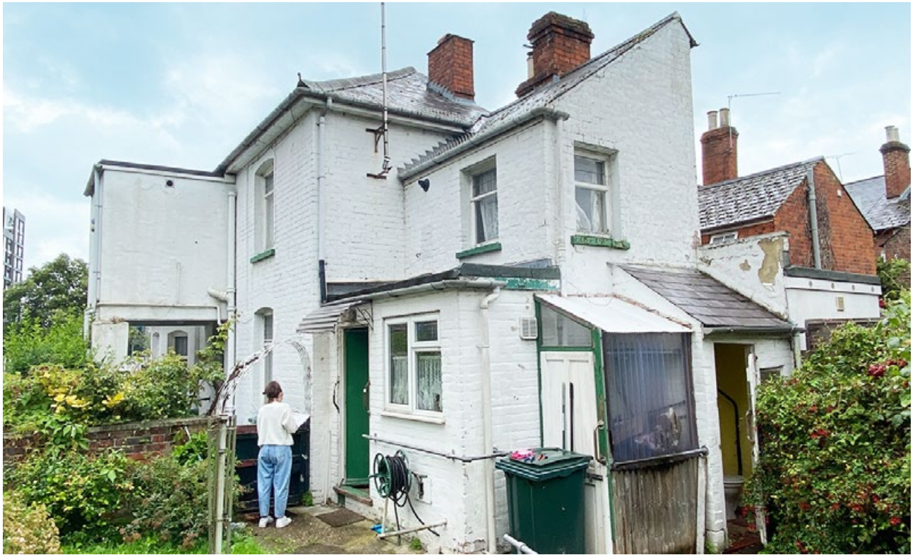
Figure 2: Existing Rear Elevation (Extracted from the Design & Access Statement ref 21009.9.1_21.11.12_DAS)
