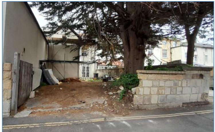
Fig 4. Rear of 24 Eldon Road. Site photo taken on 21/07/2023.
