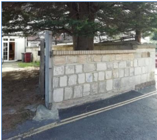
Fig 3. Rear of 24 Eldon Road. Site photo taken on 26/03/2019.
